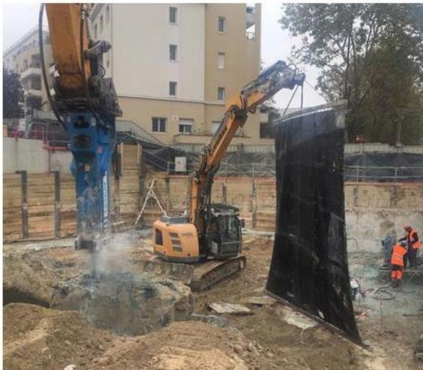
**FIGURE 16 : MISE EN PLACE DE BACHES ACOUSTIQUES GRUTABLES**
