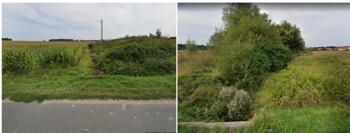
Photo 19 – Photos StreetView de la vidange des Preneux (Source : Google maps)
